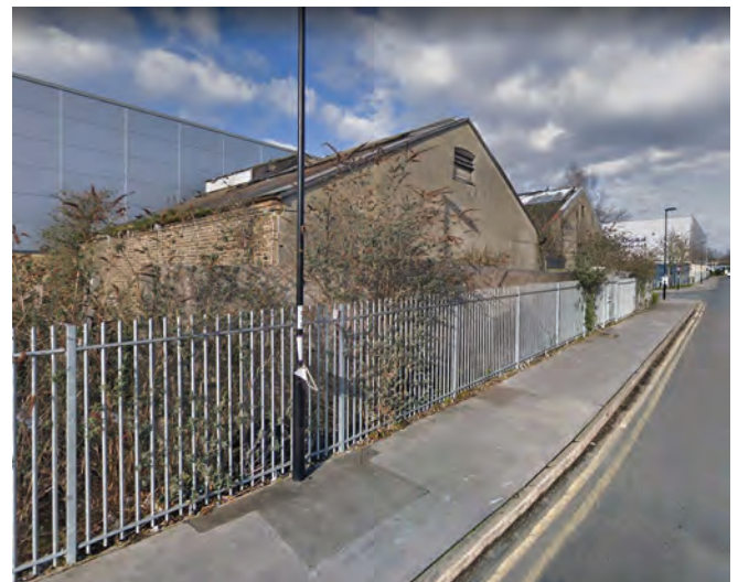
The tunnels led into the electricity substation located at the junction of Princes Way and Queensway and this is the only section of that part of the factory that survives
